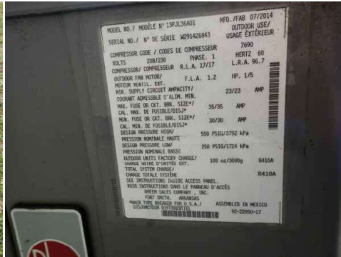
Condensing unit name plate data
