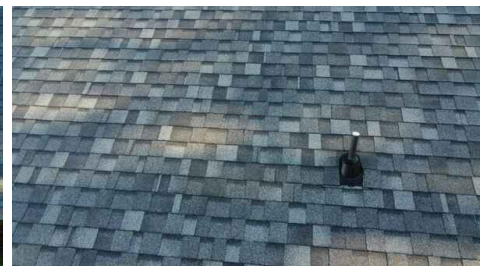
Flashing closer look
