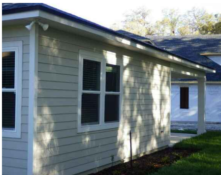
Representative exterior window image
