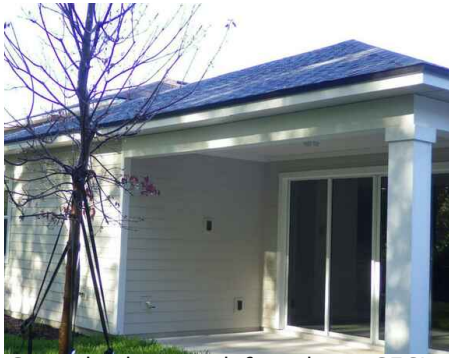
Gas valve bottom left and two GFCI electrical outlets.
