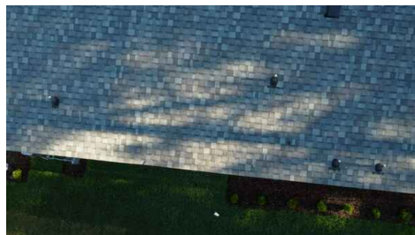
DWV flashings from another angle.
