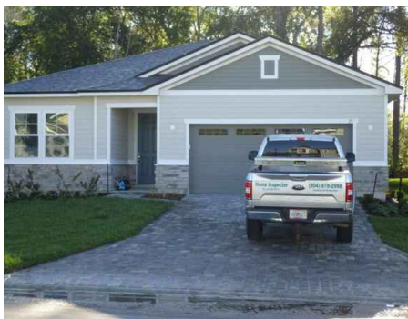
Pavers are in good condition.
