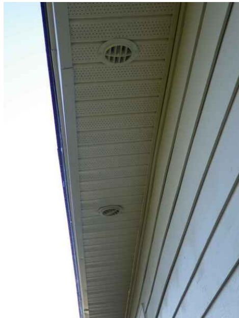
Soffit extends around the structure.
