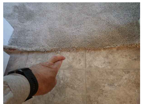
Missing threshold
