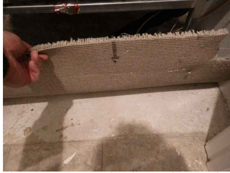
The carpet is not glued or tacked to the concrete floor. It can be easily removed.
