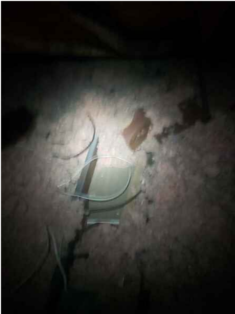
Missing insulation 1
