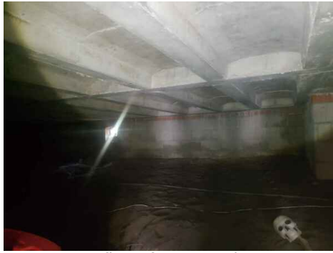
Main floor from crawlspace
