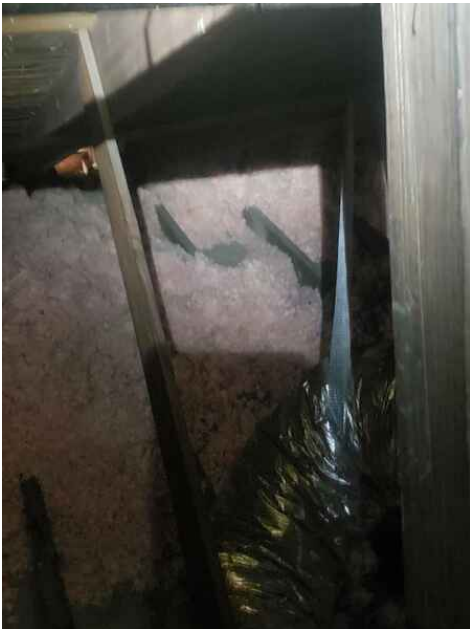
Missing insulation 4
