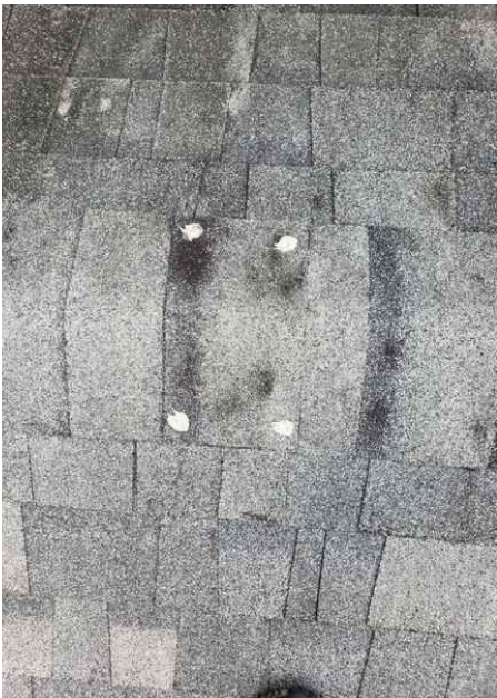
Nails sealed well
