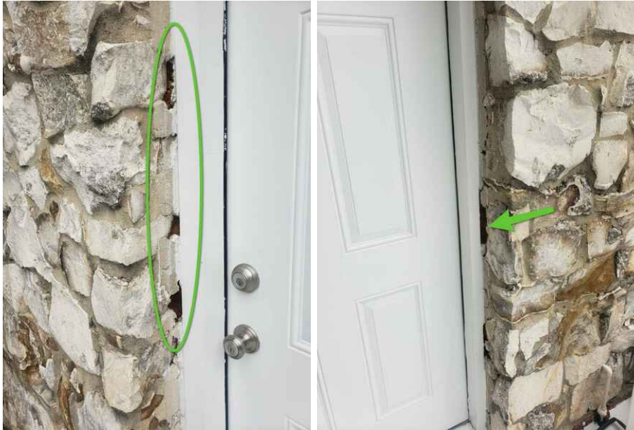
Door for pool tool storage
