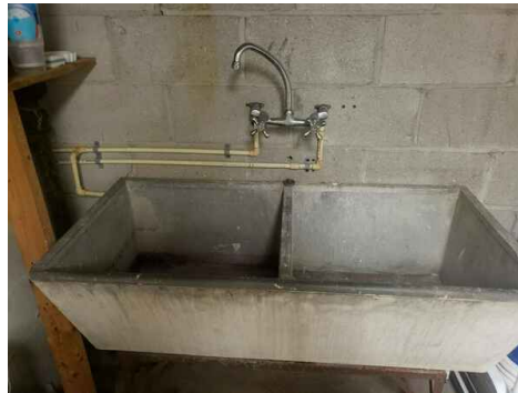
Cement laundry sink
