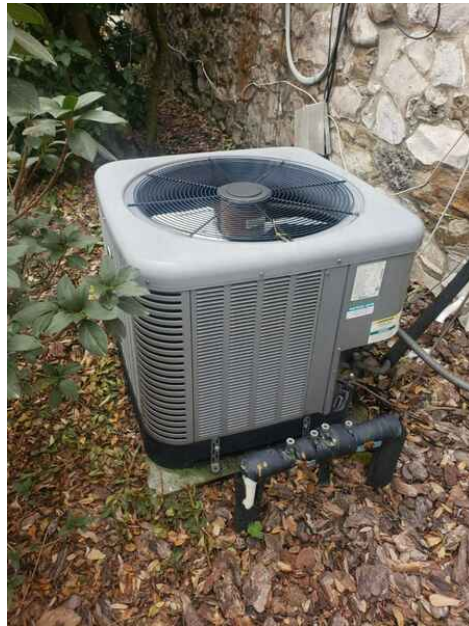
Servicing main floor
