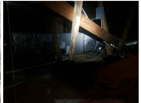
Air handling unit (main floor)
