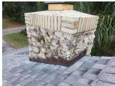
Flashing: Rubber Caulking 3
