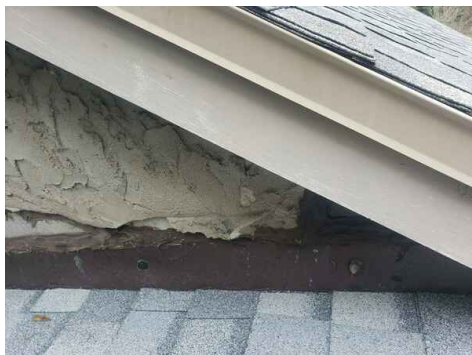
Flashing: Rubber Caulking 2
