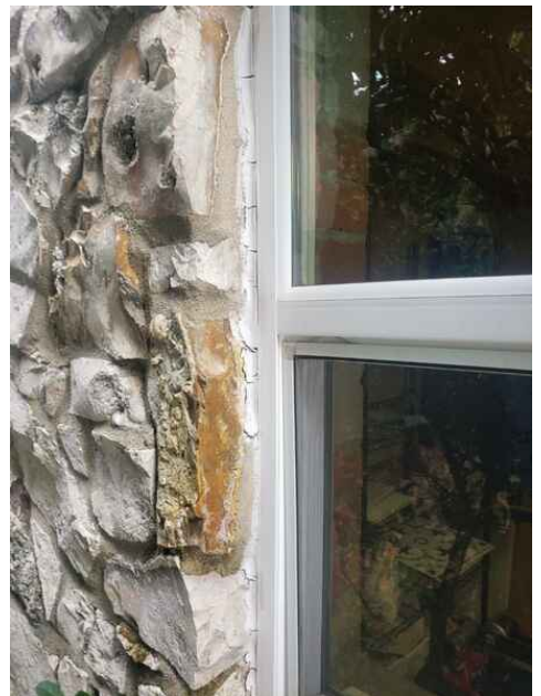
Window in back yard on north end by sewer cleanout
