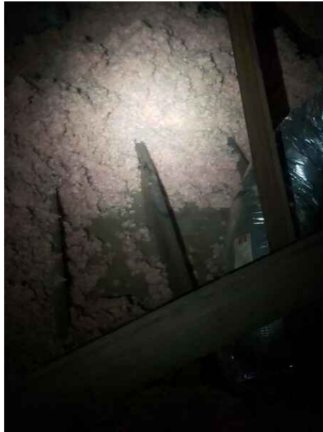
Missing insulation 2
