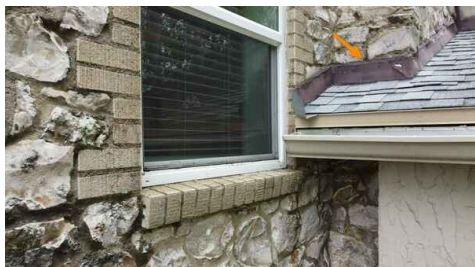
Flashing: Rubber Caulking 1
