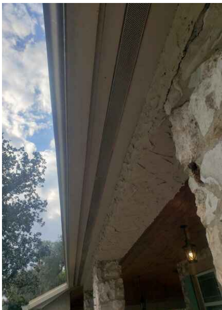
Soffit vents: Typical
