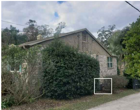
2 condensing units on north side of house
