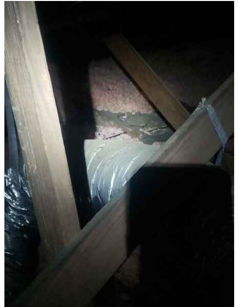
Missing insulation 3
